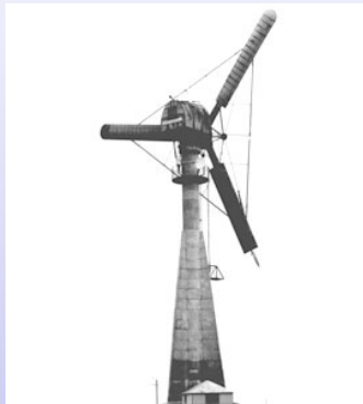
The Gedser wind turbine 1940's
