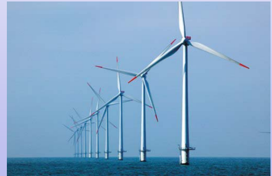
Horns Rev (DK) 80x2MW installed 2002
